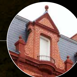
NOTABLE MANSARD ROOF
